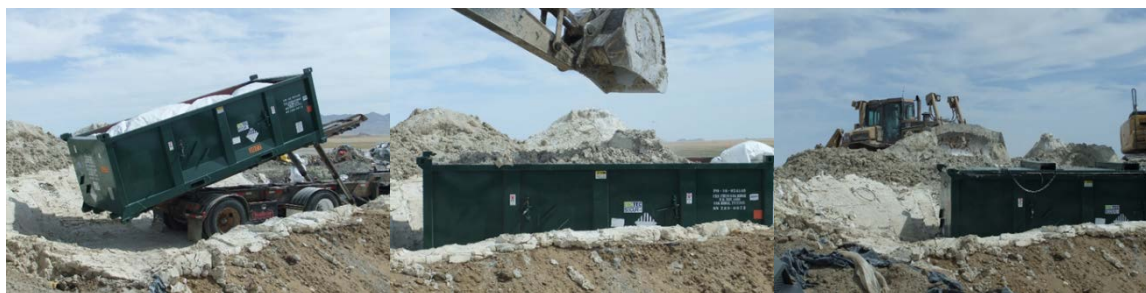
Figure 2. Macroencapsulation of COLEX Debris
