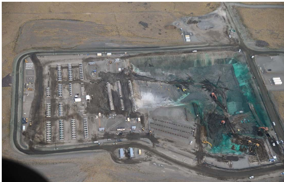
Figure G.4-4. 618-10 Burial Ground Remediation Progress 11
